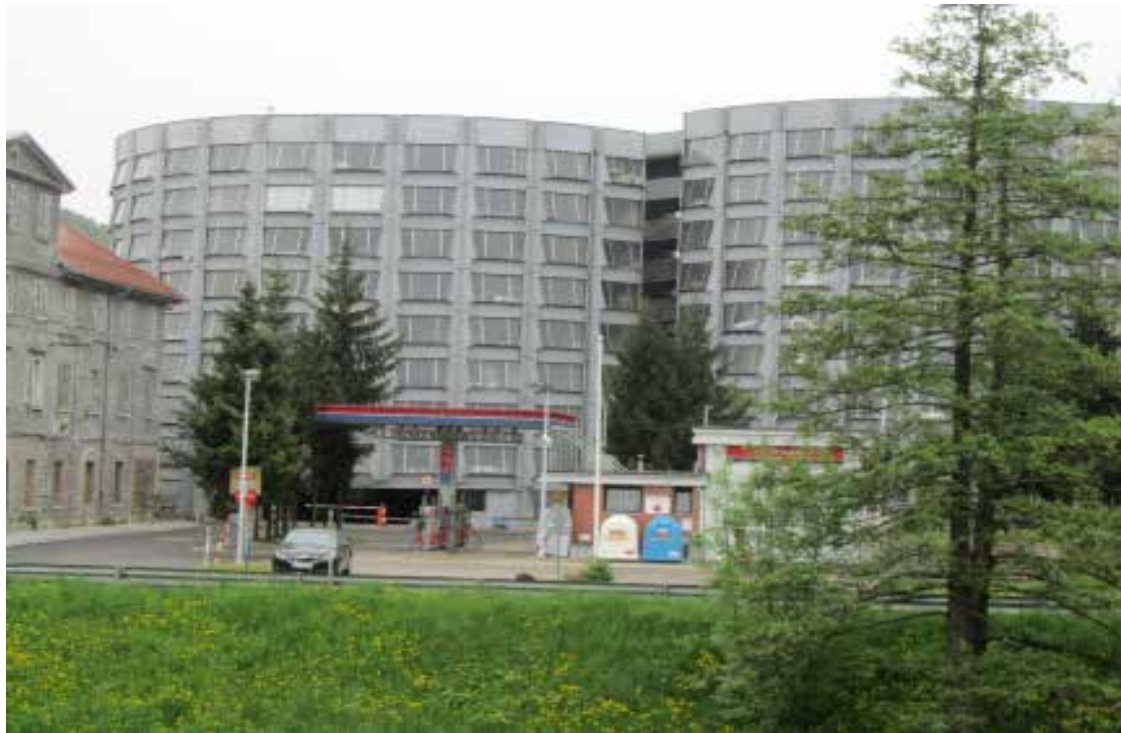
Fig 2: The Sever car park – a view from the west.
